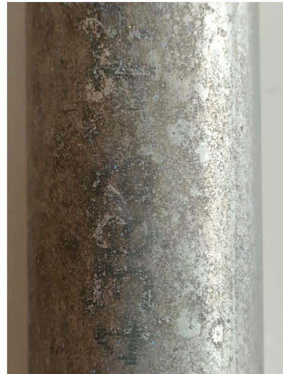
Steel pipe: rough, partially rusted
